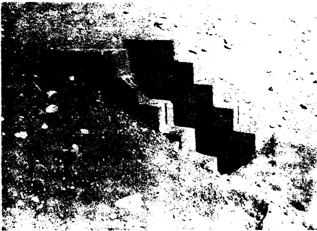
Fig. 11—Entrance to block-wall basement exit after blast.
